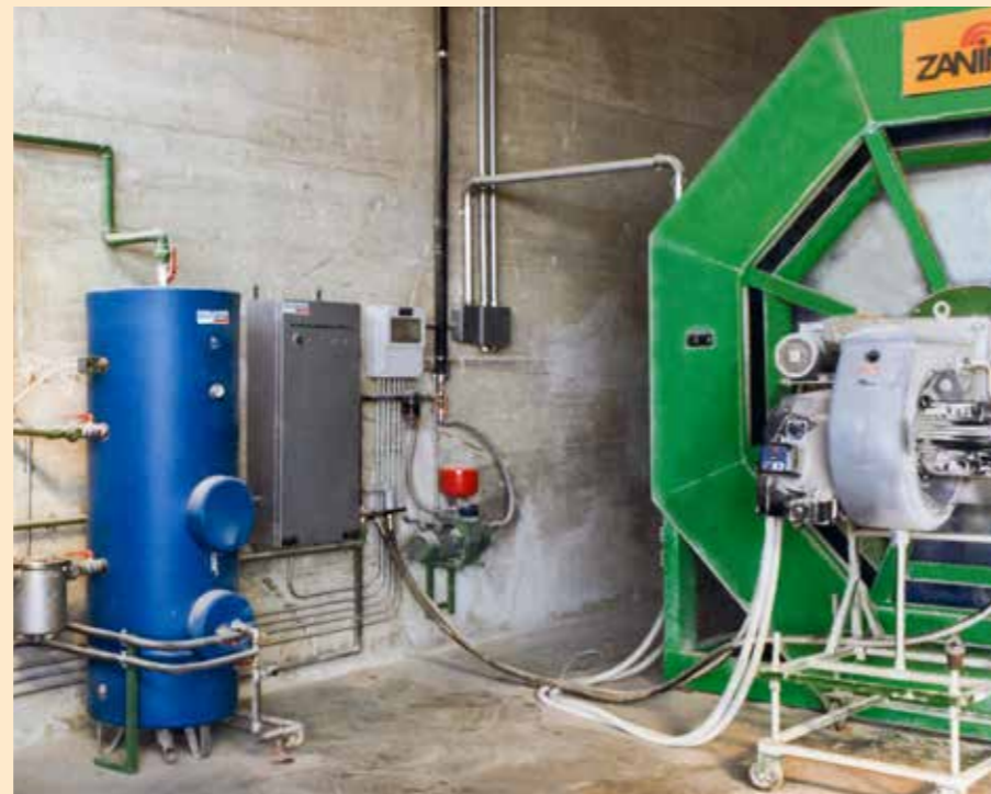
Indirect hot air generator operating with dense oil
