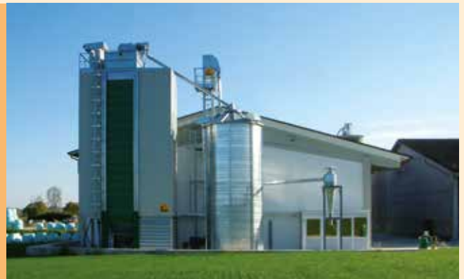
■ FIX-DRY plant with slow cooling system and horizontal magazine charging.
