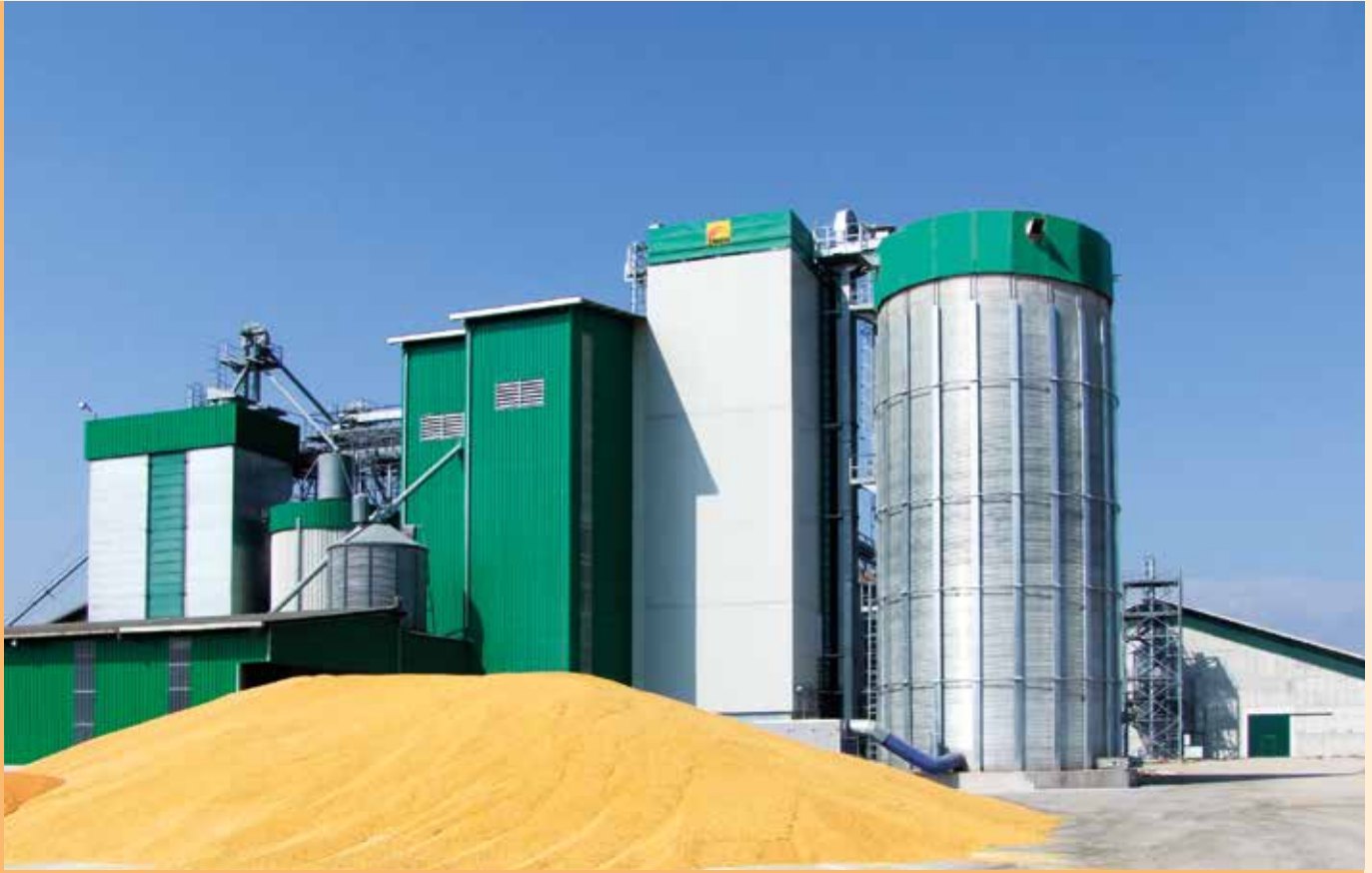
■ Cereals drying plant with CR dryer complete of slow cooler
