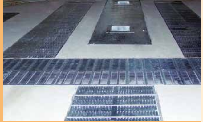
■ Ventilation conduit for silos with perforated panel
