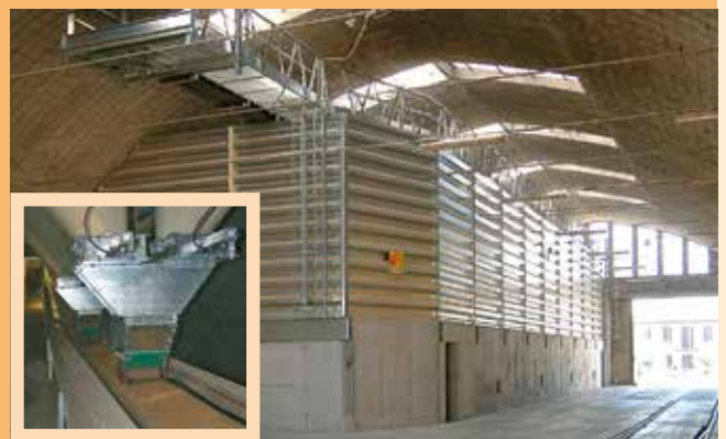
■ Square silos with discharge plant.
