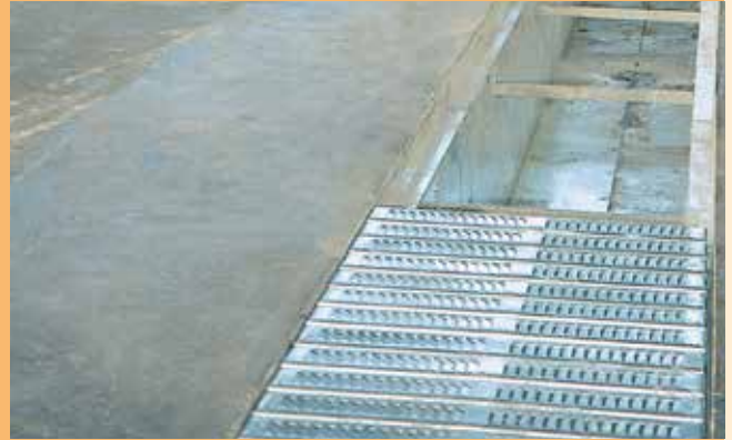
■ Floor ventilation system.
