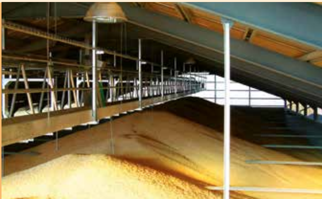
■ Horizontal store complete with conveyors.
